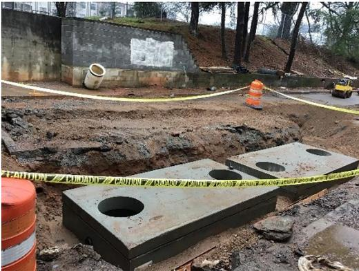
New Grease Traps Set for Sanitary Waste
